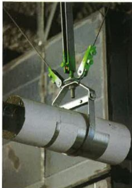
Figure 8 Solid transverse and longitudinal restraint installed at Palomar Hospital in North San Diego
