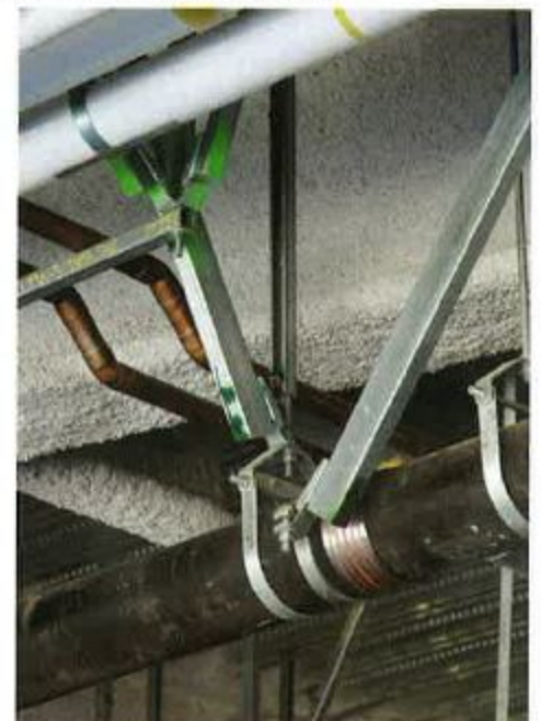
Figure 8 Solid transverse and longitudinal restraint installed at Palomar Hospital in North San Diego
